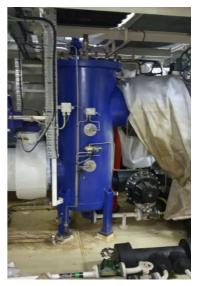
Fig. 3: BOLLFILTER type 6.18 DN500
