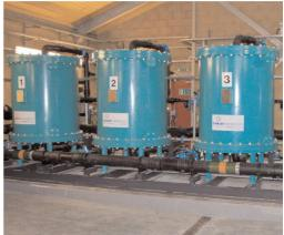
CENTRE. Skid-mounted filtration unit for installation at Severn Trent Water's Far Baulker site comprising Self-Cleaning BOLLFILTER Automatic with manual Simplex strainer as standby. BOTTOM. Typical Christ Kennicott Nitrate Removal plant.
