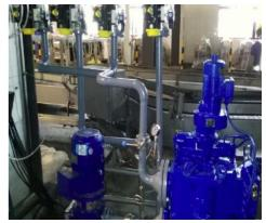
BOLLFILTER Automatic Type 6.64 at bottle washing mashine
