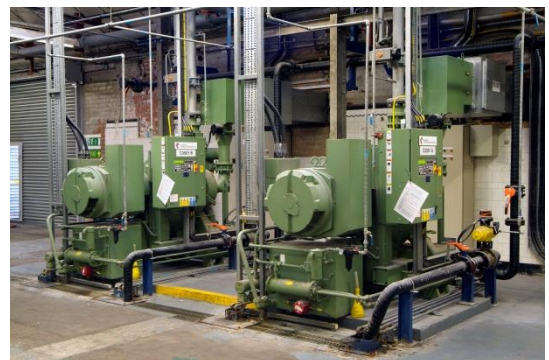
TOP. Cellulose flakes which are processed into film and filter tow. CENTRE. BOLLFILTER Automatic Type 6.18 installed to protect the Compressors. BOTTOM. Two Cooper Turbo Compressors, each with 1500 cu ft/min capacity.
