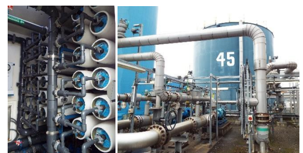
Left: SUEZ ion removal and treatment system Right: 1 micron filtered water storage ready for use
