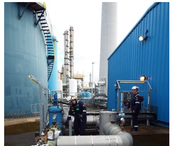
BOLLFILTER Type 6.18 DN200 and Type 1.03.2 DN200
