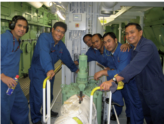
Bollfilter service training for automatic filters with the Queen Elizabeth crew in the luxury cruise liner's main engine room
