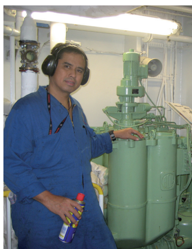
Boll 6.64.07 DN200 Automatic Lube Oil Filter
