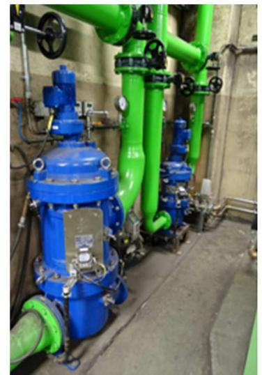
aquaBoll® automatic filter in the cooling process
