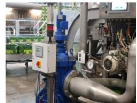
BOLLFILTER installed on crate washer
