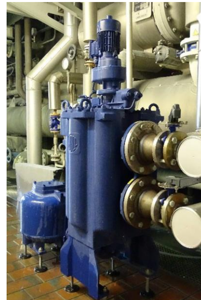
Fig. 3: BOLLFILTER automatic Type 6.64 DN125
