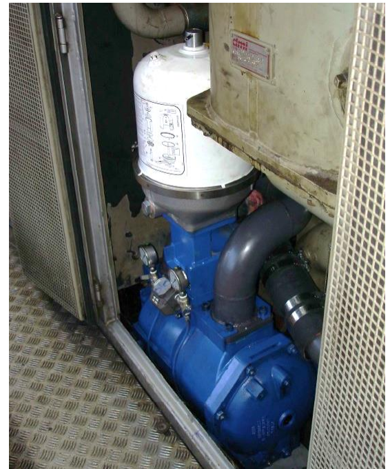
BOLLFILTER Automatic Type 6.46 DN 100 in use
