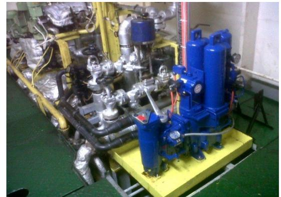
Starboard Bollfilter main engine fuel filter type 6.72.1
