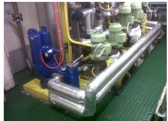
Port Bollfilter main engine fuel filter type 6.72.1
