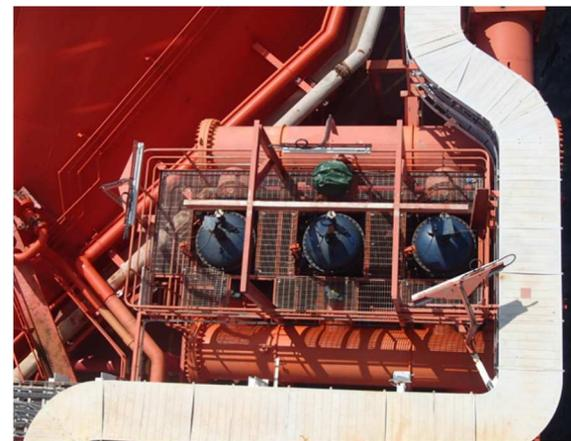
Birdseye view of the 3 BOLLFILTERs Automatic Type 6.18 DN 800
