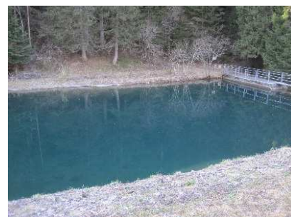
Picture 2: Reservoir during the summer months
