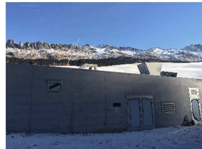
Picture 1: Exterior view of the pump station
