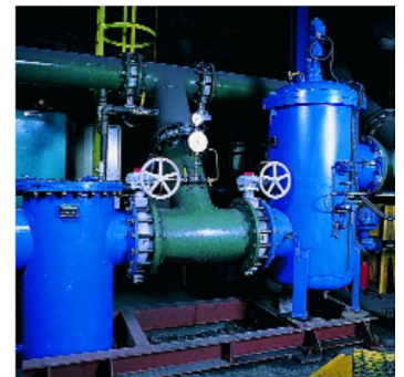
Installation of BOLLFILTER Automatic Type 6.18
