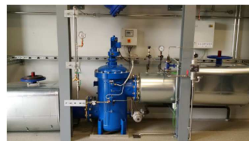
Filter in operation
