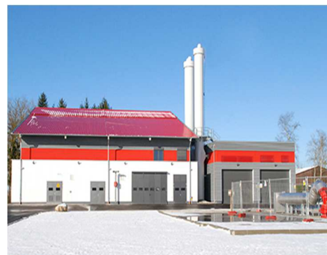
Heating plant Ismaning
