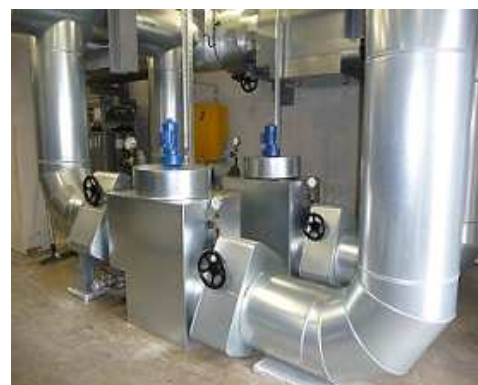
Filter in parallel operation, with isolation
