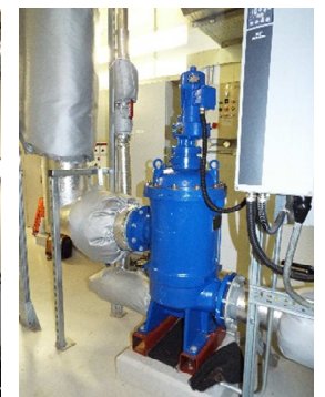
Right: BOLLFILTER 6.18 in Operation
