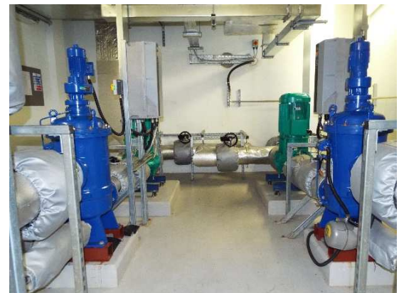
Two x BOLLFILTER Type 6.18 Filters in parallel
