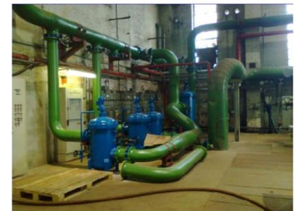
Fig. 2: Installation of BOLLFILTER system with pre-filter (background)
