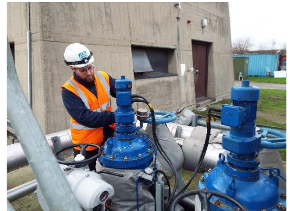
2 x BOLLFILTER Type 6.18 DN150 Final Effluent Filters
