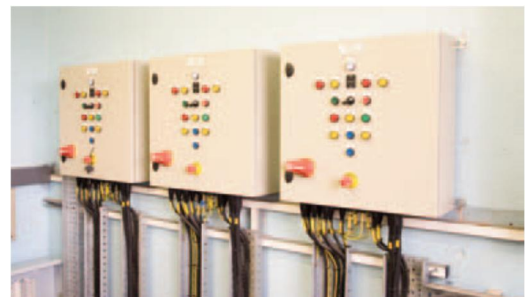
TOP. Typical Memcor Continuous Ultrafiltration System. CENTRE. BOLLFILTER System comprising three Self-Cleaning BOLLFILTER Automatic Type 6.18 SUC. ABOVE. Each filter has a control system with alarm linked to a remote monitoring centre.
