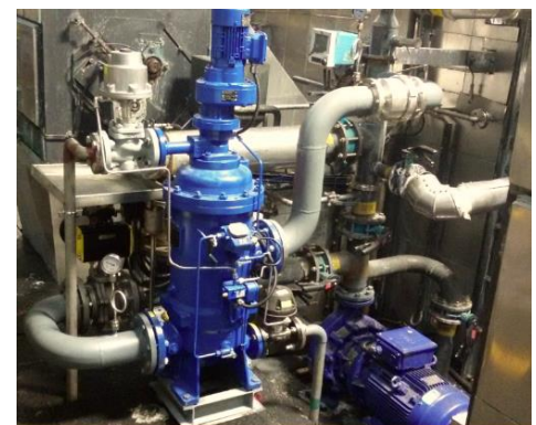
1 Skid unit with BOLLFILTER Automatic Type 6.19 DN 100 installed at ABInBev Suqian plant
