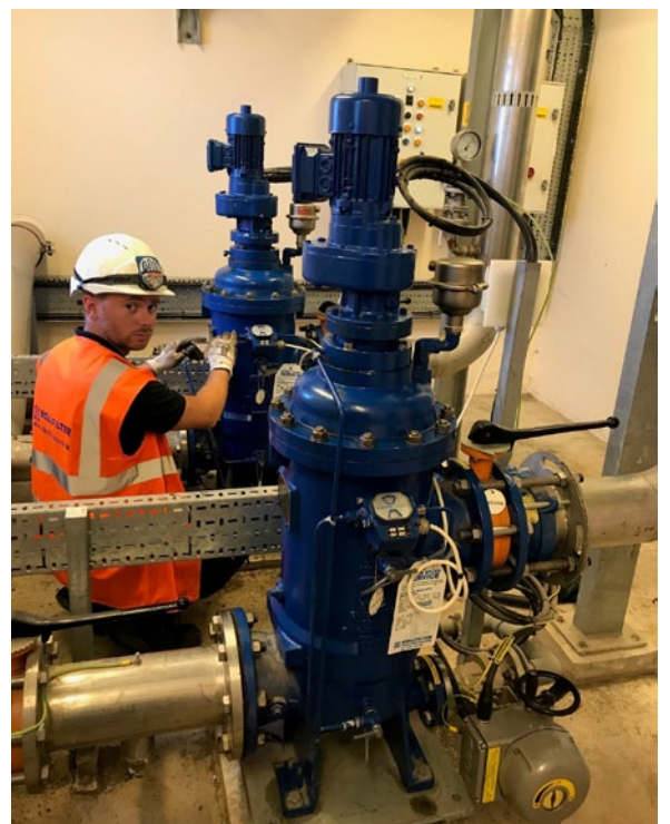
Chris Ludlow, Service Engineer, working on site
